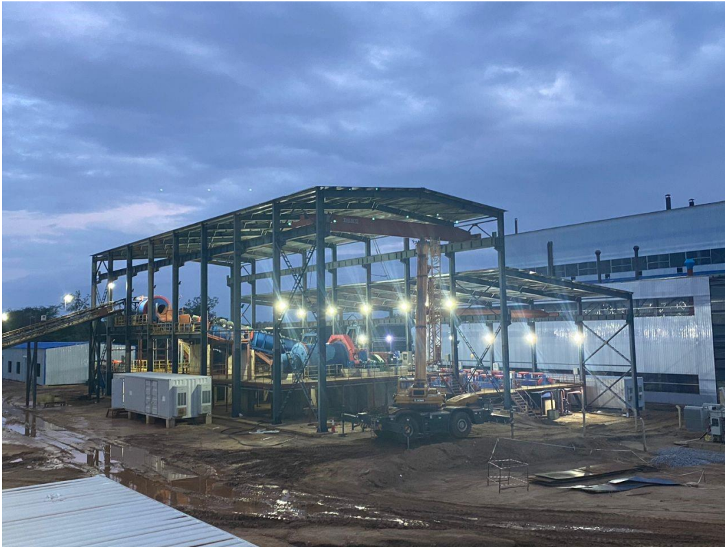
Figure 2: Concentrator Building after connection to Tanesco Power.
