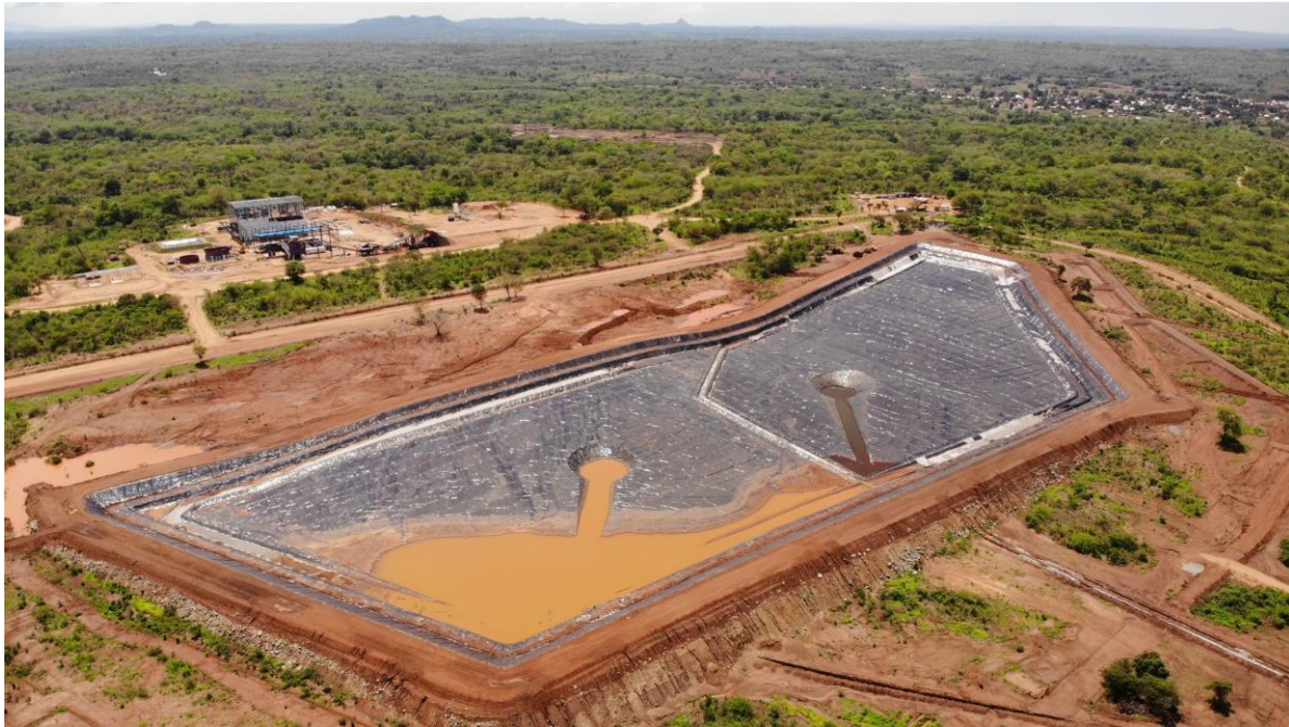
Figure 2: HDPE lining of the TSF at the end of December 2023.
