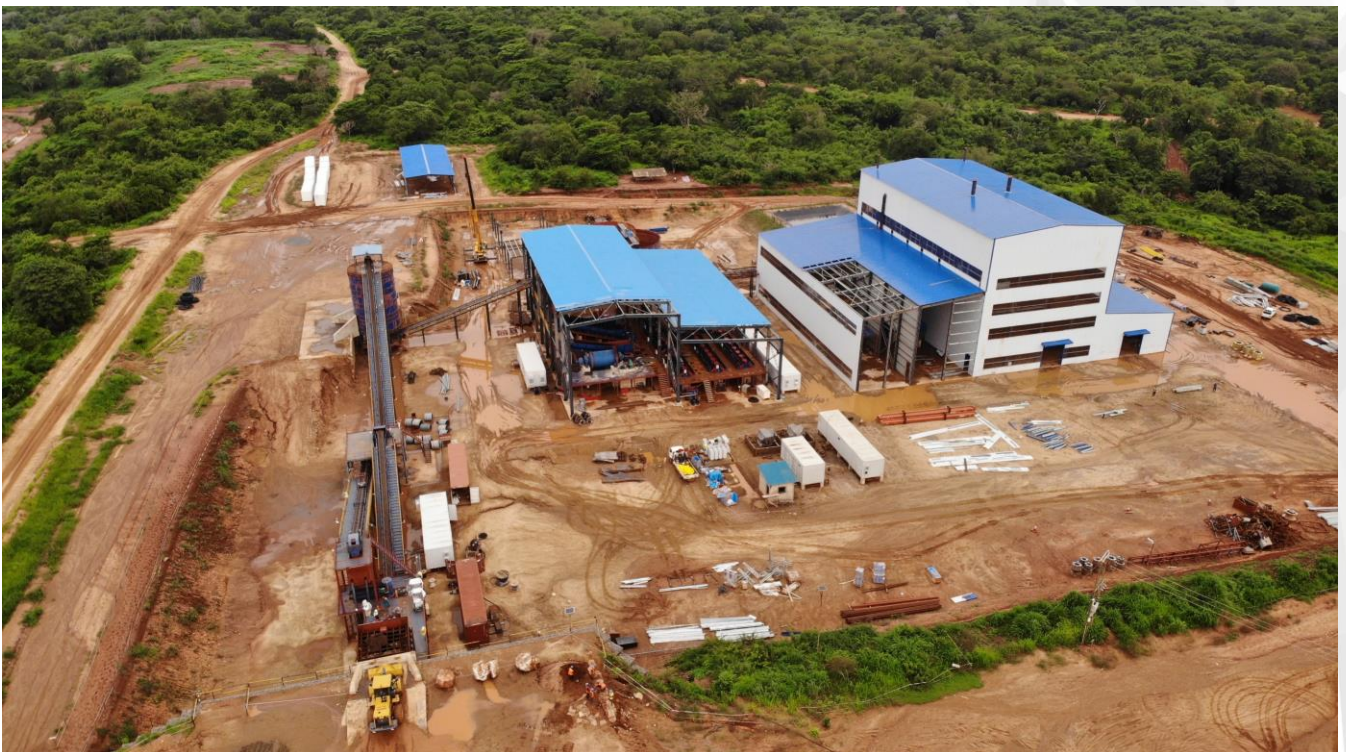
Figure 1: View of the Processing Plant in January 2024.
