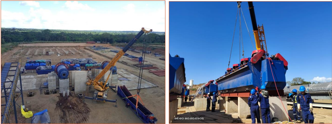
Figure 3: Lift of the secondary spiral classifier (left) and flotation cells (right).
