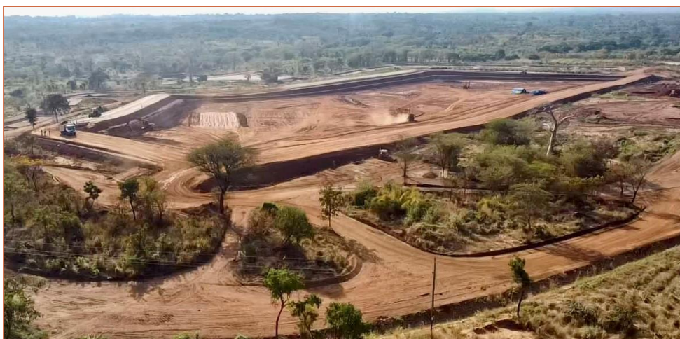
Figure 1: Oblique view of the TSF from the southwest as at the end of June. Note the compaction of the clay layer on the retaining wall on the northwestern side of the TSF (top left side) and the preparation of the basin for the HDPE liner to be installed in the third quarter.
