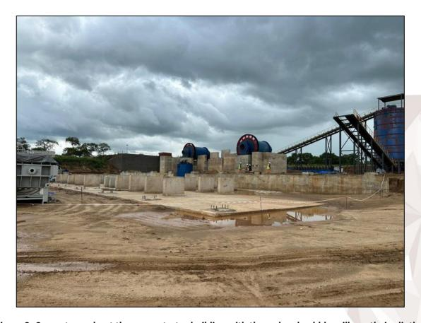
Figure 2: Concrete works at the concentrator building with the rod and pebble mills on their plinths.
