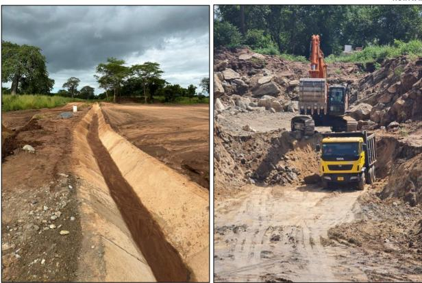
Figure 1: Portion of the solution trench around the TSF (left) and mining of waste rock for the TSF retainer walls in March 2023 (right).
