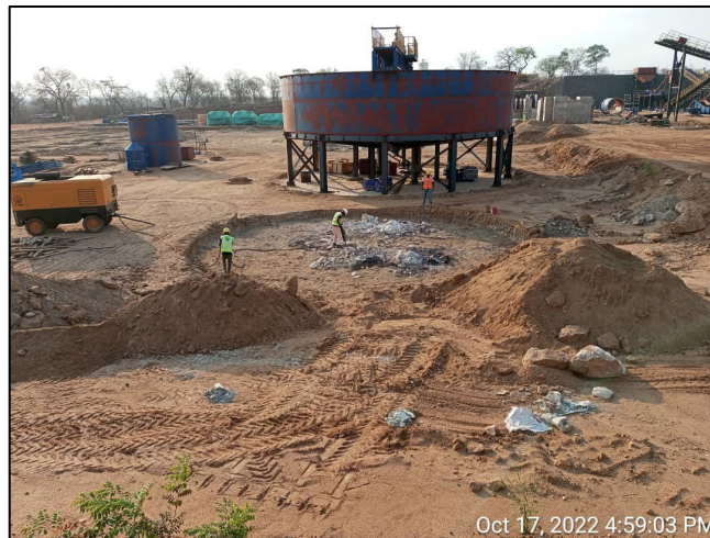
Figure 2: Mechanical installation of the make-up water tank (left) and thickener (right).
