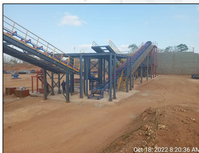
Figure 1: Mechanical installation of the crushing circuit (left) and Conveyors 1,2 & 3 (right). *Note that conveyor belting will be installed closer to commissioning.
