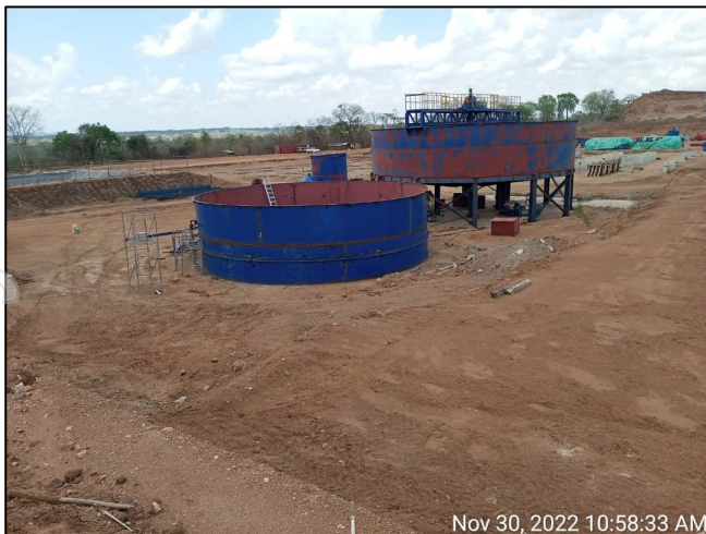
Figure 2: Mechanical installation of the make-up water tank (left) and thickener (right).
