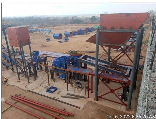
Figure 1: Mechanical installation of the crushing circuit (left) and Conveyors 1,2 & 3 (right). *Note that conveyor belting will be installed closer to commissioning.
