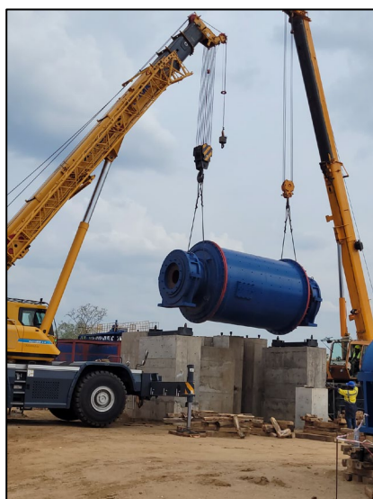
Figure 3: Dual lift of the rod mill (left) and the installation team after the lifts and mechanical installation of the rod and pebble mills (right).
