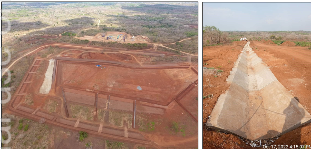
Figure 3: TSF as at the end of August 2022 with the first lift embankment wall (left) and stormwater drainage channels around the TSF (right).
