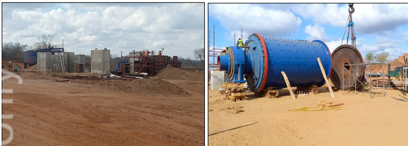
Figure 4: Concrete plinths for the rod and pebble mills (left) and the assembly of the pebble mill (right).
