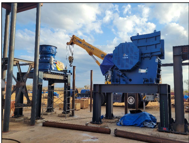
Figure 1: Installation of the jaw and cone crushers (left) and conveyors 1, 2 and 3 together with the 18m high fine ore bin (right).
