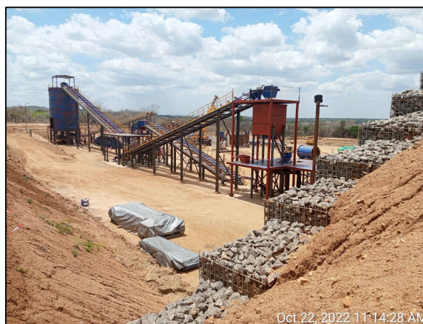
Figure 1: Installation of the jaw and cone crushers (left) and conveyors 1, 2 and 3 together with the 18m high fine ore bin (right).
