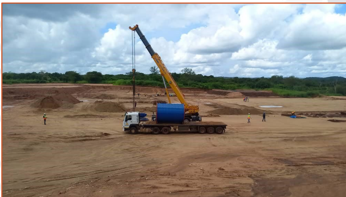
Figure 1: Offloading of the rod-mill on site using the Lindi Jumbo 55 tonne mobile crane.
