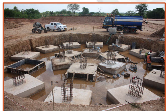
Figure 4: ROM Retaining wall (left) and thickener foundations (right).
