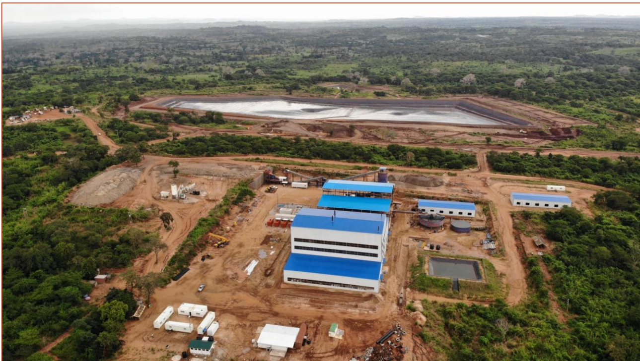
Figure 2: Aerial view from the south of the Lindi Jumbo processing plant with the TSF in the background.
