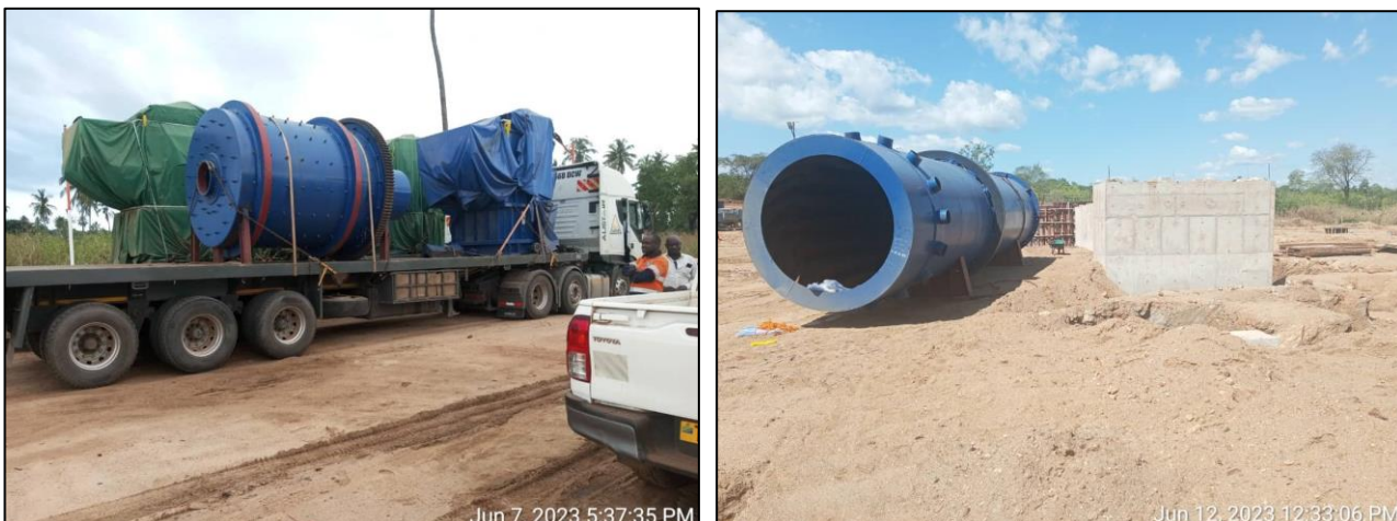
Figure 2: Drum Scrubber and attritioning mills on site (left) and two sections of the rotary drier in temporary laydown near the mounting plinths (right).
