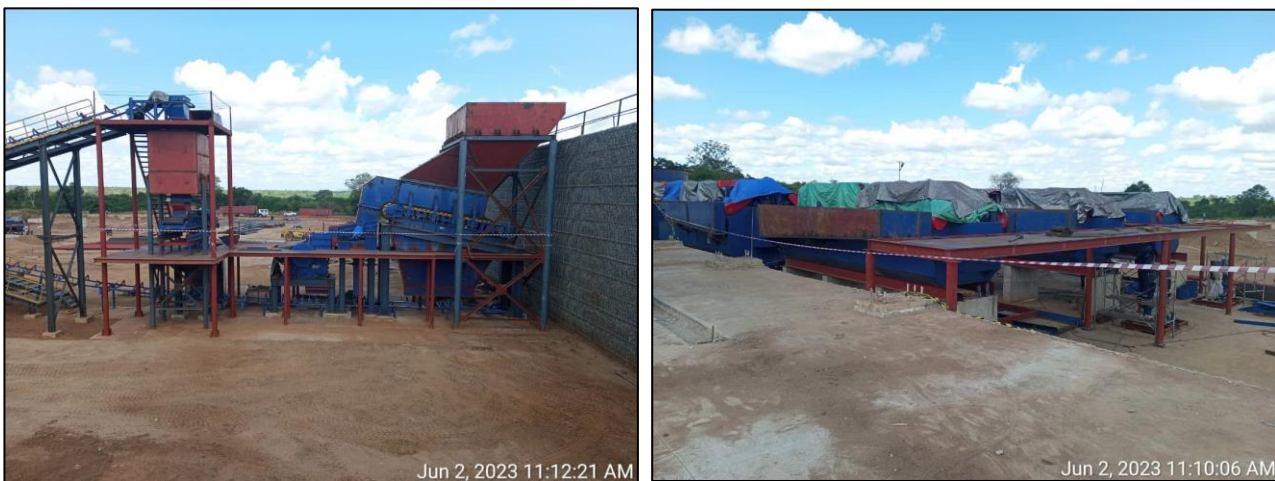
Figure 2: Mechanical completed crushing circuit (left) and the platforms around the flotation circuit (right).
