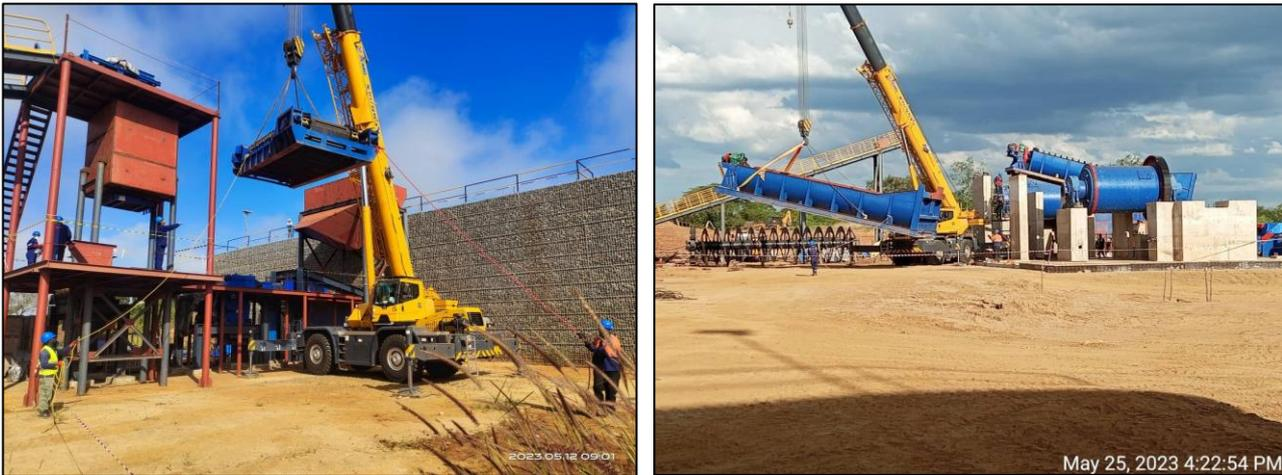
**Figure 2: Installation of the apron feeder (left) at the primary crusher and of the primary spiral classifier (right).**
