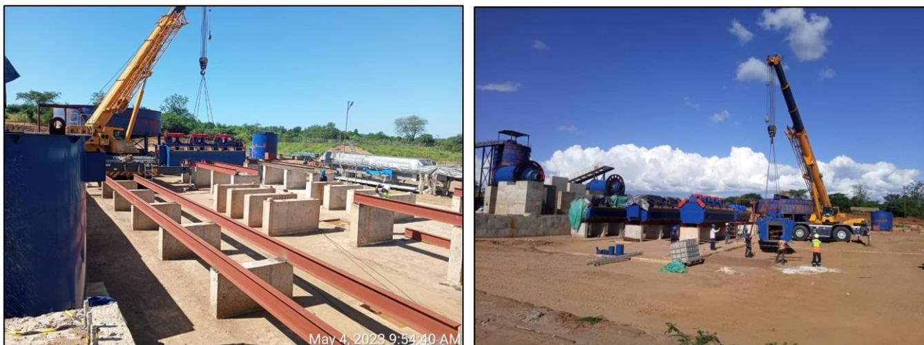
**Figure 2: Lifts of the flotation cells onto their plinths on the lower section of the concentrator building. Note the lift of the last flotation cell in the picture on the right.**
