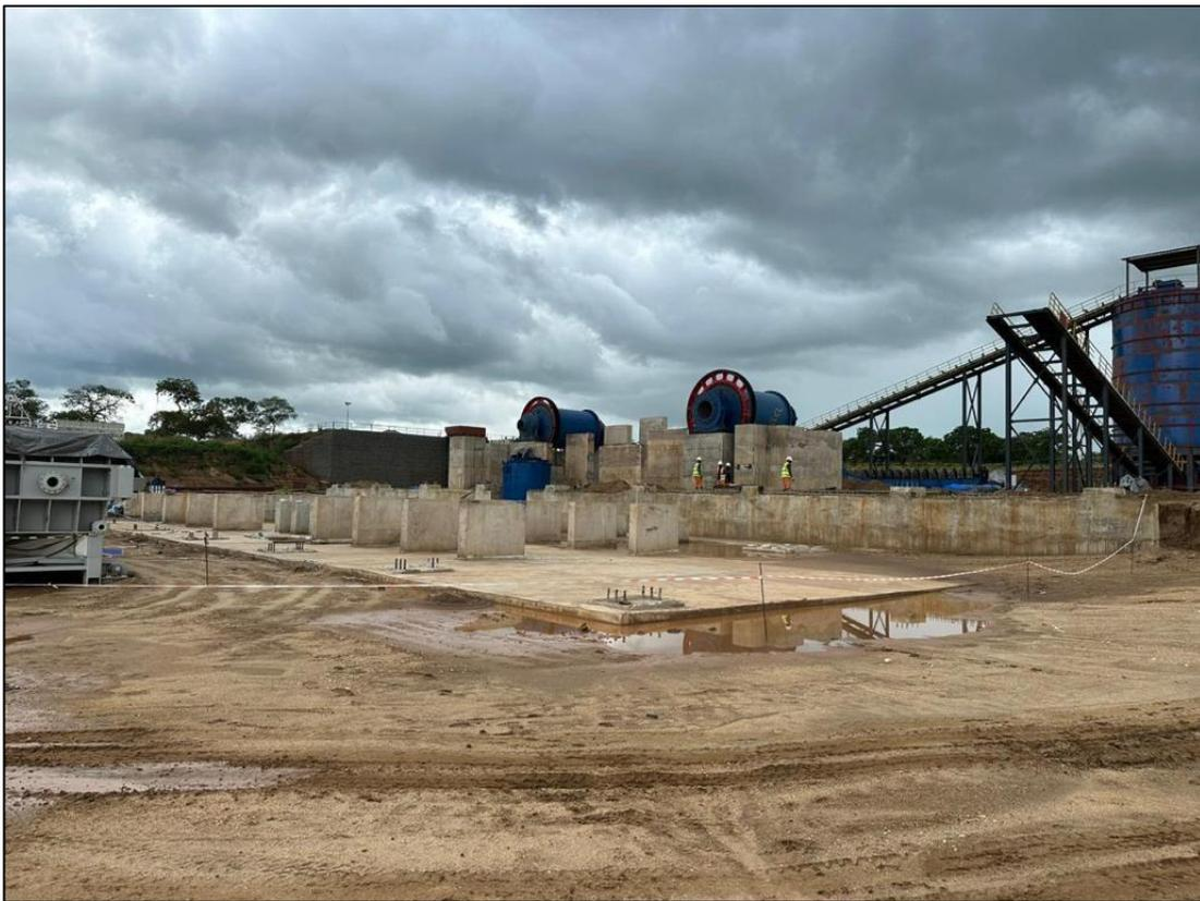
**Figure 2: Concrete works at the concentrator building with the rod and pebble mills on their plinths.**
