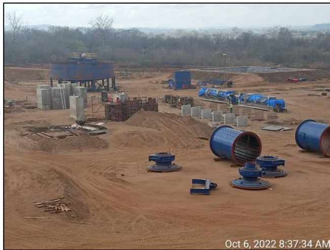
Figure 3: Concrete foundations for the rod, pebble mill and first bank of floatation cells (left) and the large spiral classifier with mill foundations (right). * Note the shells, bearings and ends of the rod and pebble mills laid out for assembly and installation.
