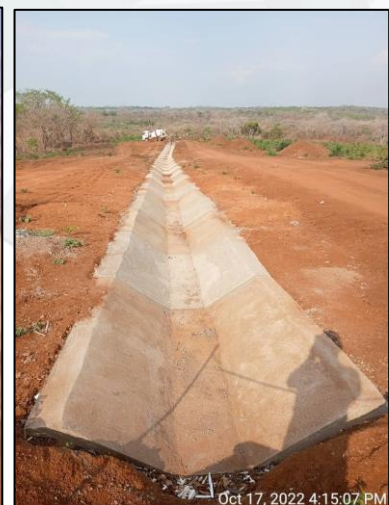
Figure 4: TSF construction progress (left) and the continuation of the minor concrete works through the construction of the stormwater drainage (right).
