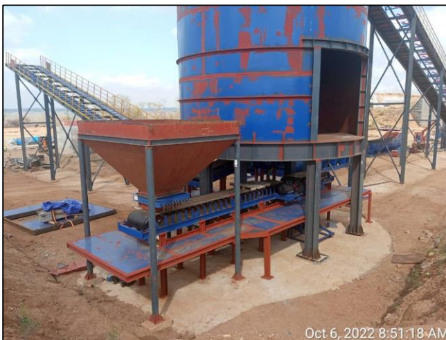
Figure 2: Mechanical installation of the fine-ore bin and feed conveyor (left) and thickener (right). * Note the preparations for the foundations in the foreground of the make-up water tank alongside the thickener.
