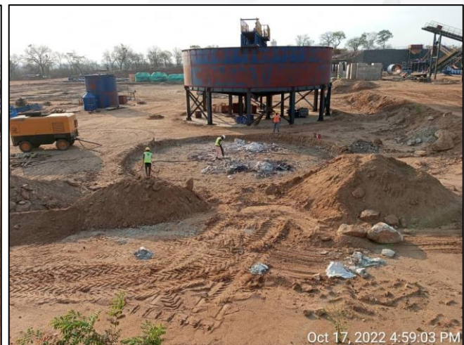
Figure 2: Mechanical installation of the fine-ore bin and feed conveyor (left) and thickener (right). * Note the preparations for the foundations in the foreground of the make-up water tank alongside the thickener.
