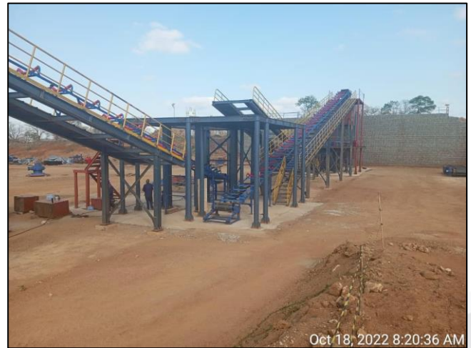
Figure 1: Mechanical installation of the crushing circuit (left) and Conveyors 1,2 & 3 (right). *Note that conveyor belting will be installed closer to commissioning.
