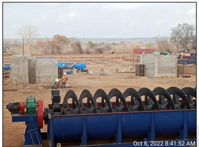
Figure 3: Concrete foundations for the rod, pebble mill and first bank of floatation cells (left) and the large spiral classifier with mill foundations (right). * Note the shells, bearings and ends of the rod and pebble mills laid out for assembly and installation.
