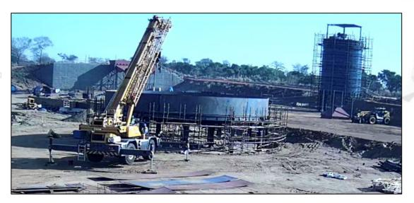
Figure 1: Construction at the Lindi Jumbo Mine. The thickener is in the foreground with the fine-ore bin in the background.
