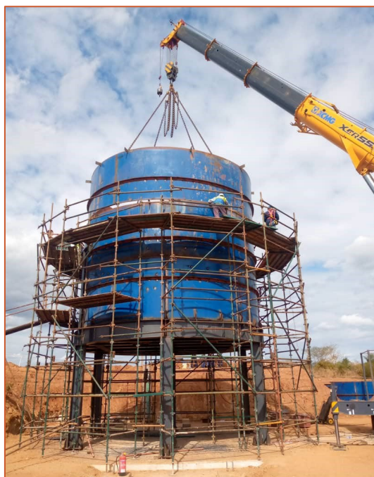
Figure 6: Assembly of the fine-ore bin. Once completed the structure will be 18m high.
