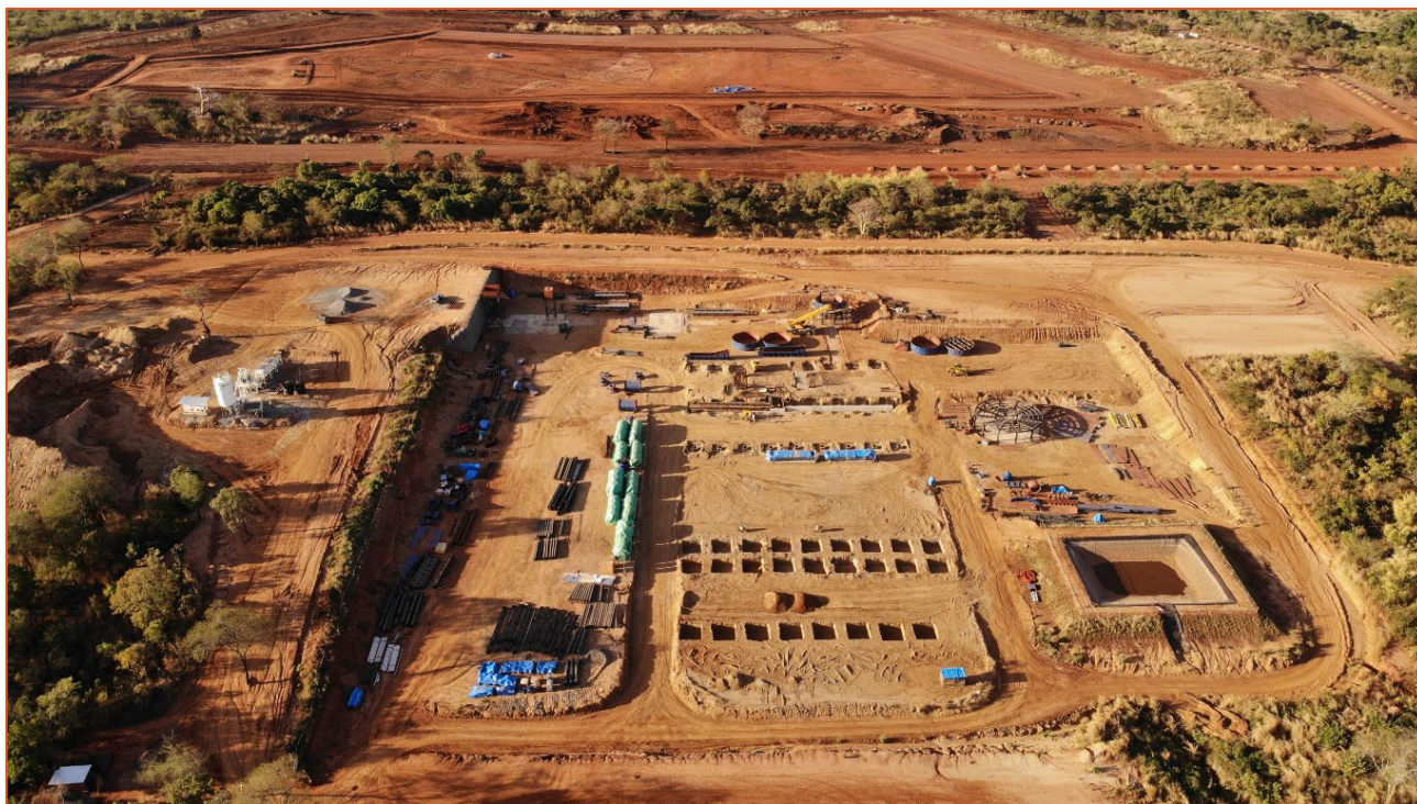
Figure 5: End of June 2022, view from the south of the processing plant area with the TSF in the background. Development of foundations for the drying, screening and packaging building can be seen in the foreground.
