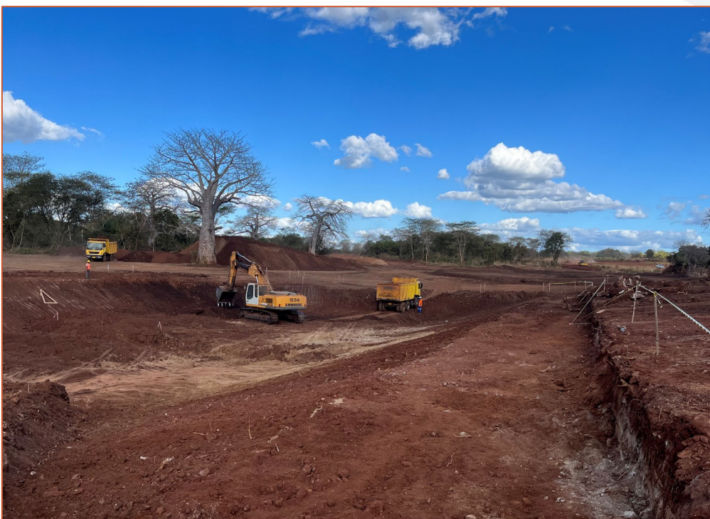
Figure 4: Excavation and shaping of the return water sump at the distal end of the TSF.
