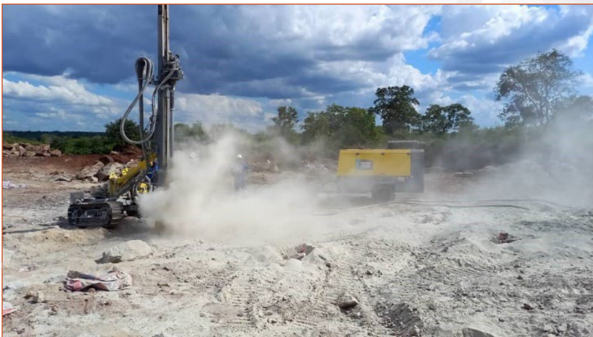
Figure 7: Drilling in preparation of the first blast.
