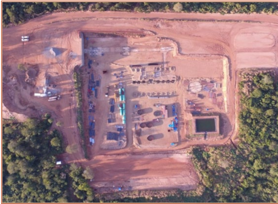
Figure 2: Top view of the processing plant area. Numerous pieces of equipment visible including the floatation cells, filter presses, crushers, screw classifiers, fine ore bin sections and laydown of the structural steel components.
