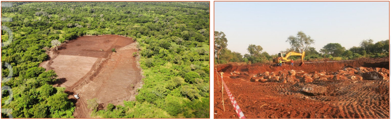
Figure 6: Starter pit pre-strip. The area is approximately 700m to the west of the Processing Plant area. Approximately 0.30 to 1m of clay rich saprolitic waste material has been used in the construction of the TSF.
