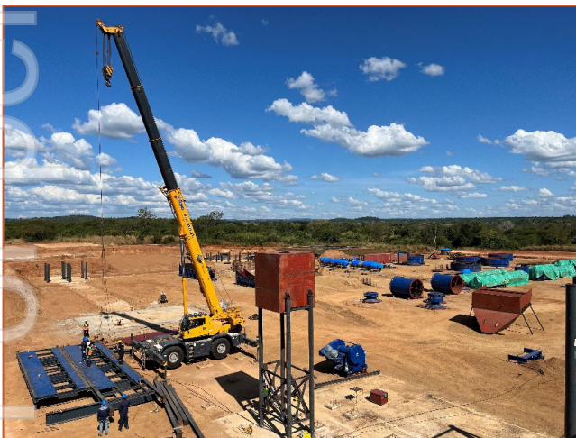
Figure 5: Steelwork construction on site using the Lindi Jumbo 55-ton crane (left) and transport of an assembled section of the fine-ore bin for installation (right).
