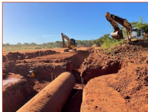
Figure 1: Oblique view from the south of the TSF. Clay filled cut-off keys around the TSF footprint are clearly visible (left). Excavation of the stormwater cut off trench at the TSF (right).
