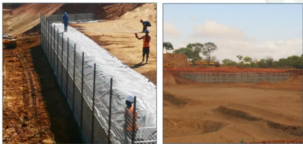
Figure 4: ROM Retaining wall (Terra Trel wall) as of 06 December 2021.
