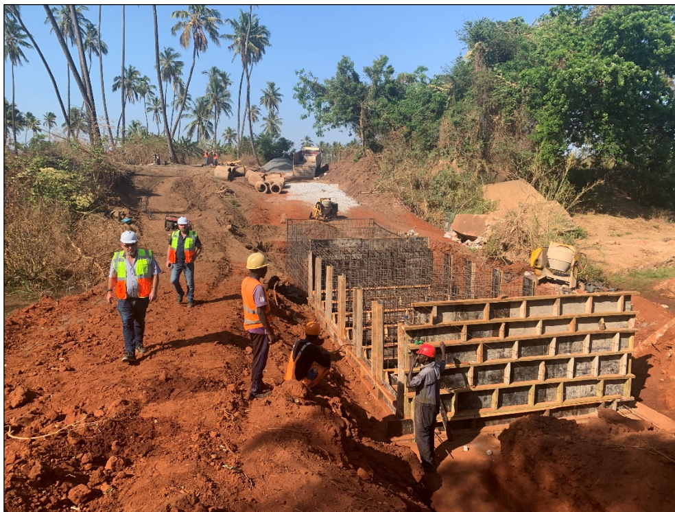
Figure 3: Allan Mulligan (COO) and Bruce White (PM) inspecting the construction by TNR of the Tanroads designed Low Water Bridge over the stream near Ruangwa.
