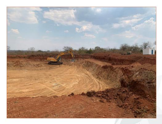
Figure 2: Terracing and levelling of the Processing Plant area.
