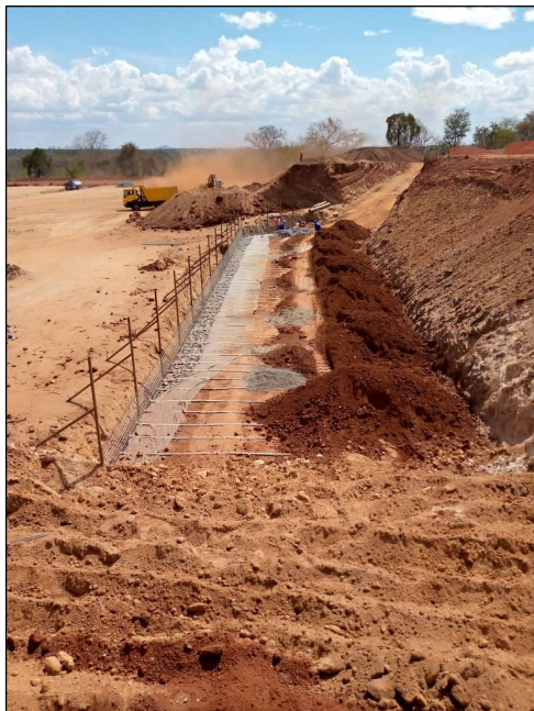
Figure 2: Start of the ROM Retaining Wall (left) and plant terracing (right) in November 2021.
